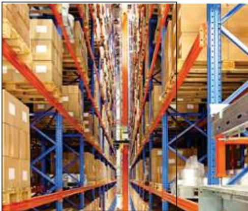
Stacker Crane ASRS
