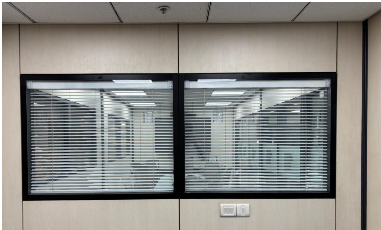
Motorized Venetian blinds seamlessly integrated into a Double Glass Frame.
